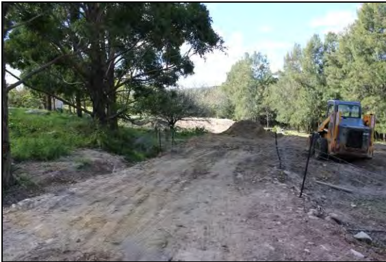
Photograph 28: Cleared land at Lot 1059
