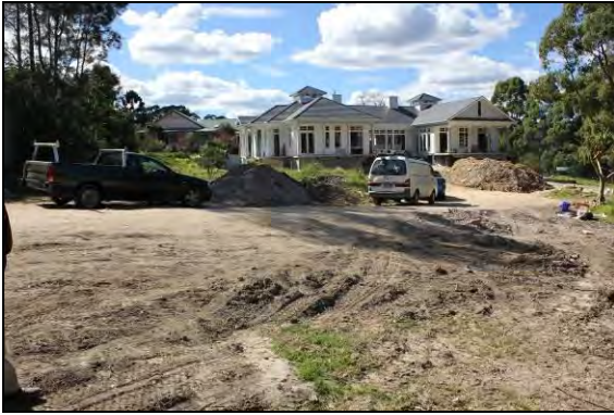
Photograph 26: Cleared land at Lot 1059
