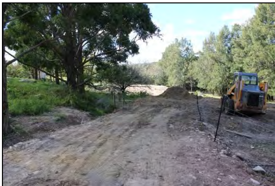
Photograph 3: Cleared land at Lot 1059
