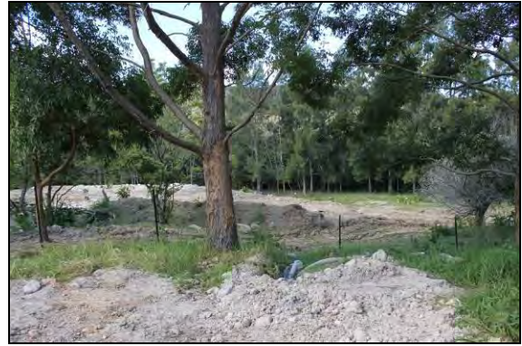
Photograph 27: Cleared land at Lot 1059
